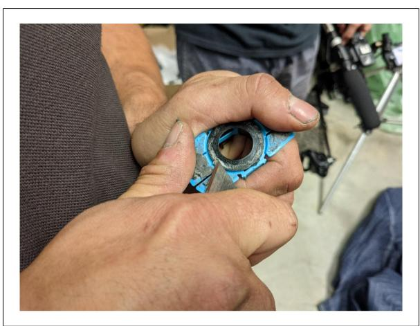
53. Remove remnant adhesive from the face of the sensor housing, using a utility knife and / or solvents.
